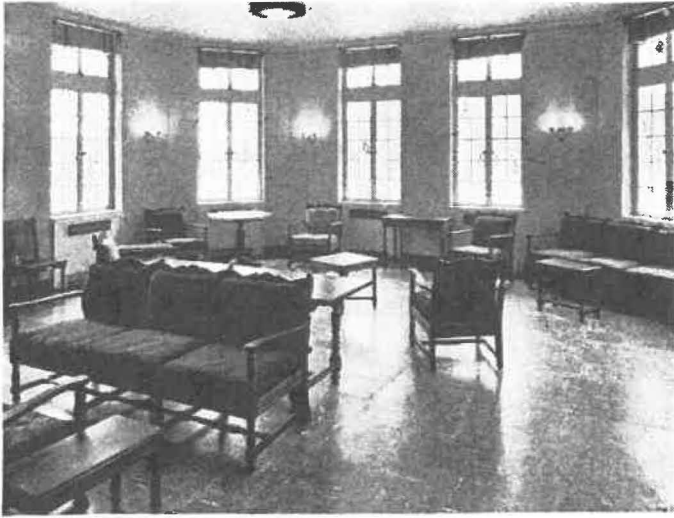
Detention Home Public Parlor
